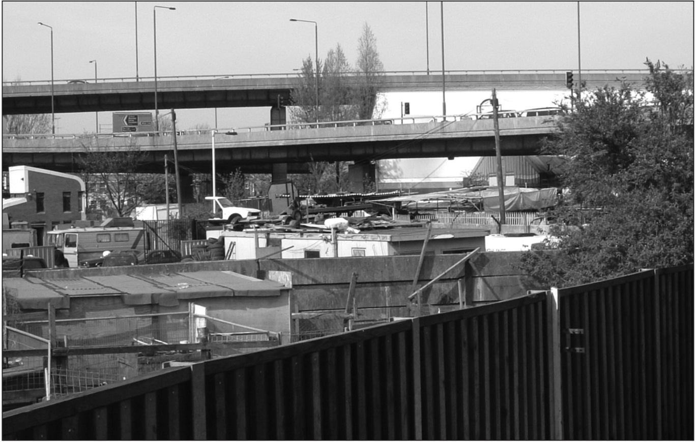
Figure 4.1: Example of the impact of poor design
